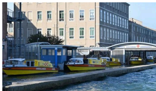
Entrance from Fondamente Nove Jona Reception
